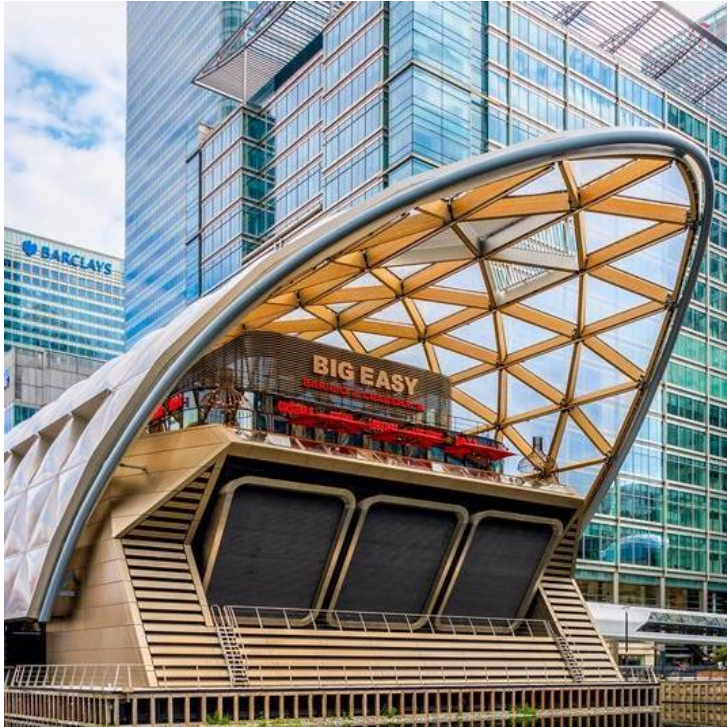
Crossrail Station Canary Wharf - Great Britain
