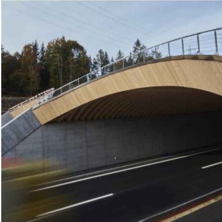
Wildlife crossing bridge - Switzerland
