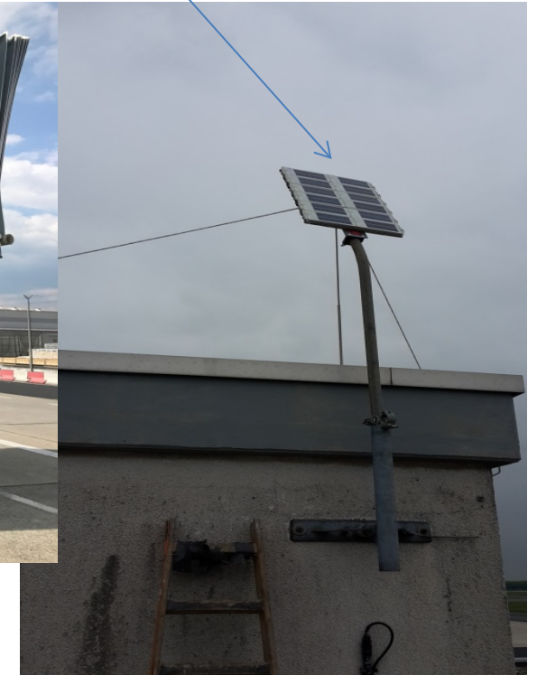
Gateway without power cord by solar energy harvesting
